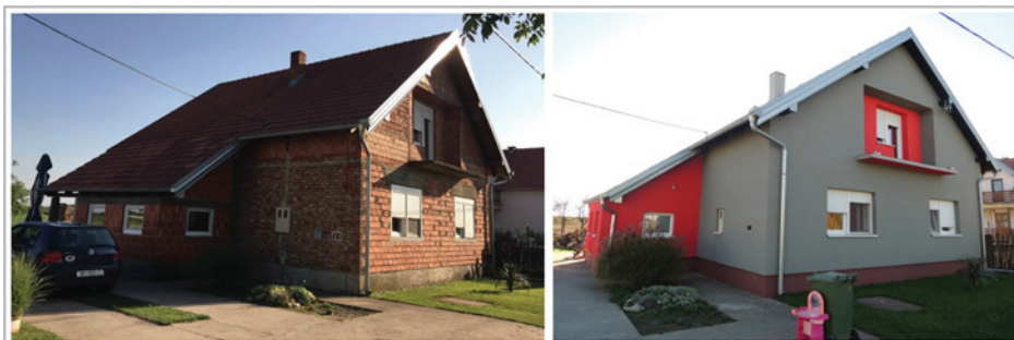
Figure 5. Example of a family house before and after refurbishment – hose has moved from energy class E to energy class C (160 kWh/m 2 -> 54,5 kWh/m 2 )
